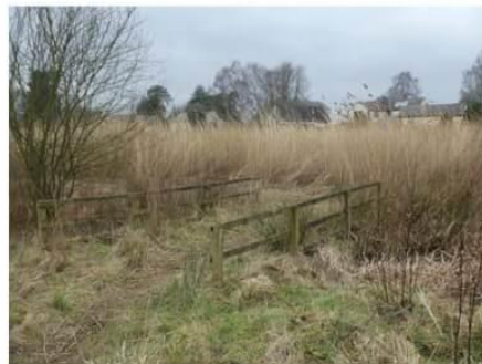
The cleared bridge leading to the reed bed
